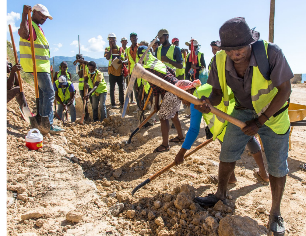
Photo: Community rubble clearance in Chardonnières, Haiti, after the 2021 earthquake.
